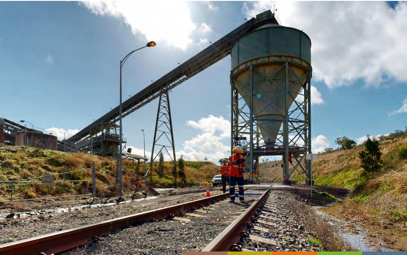
Track inspection, New South Wales
